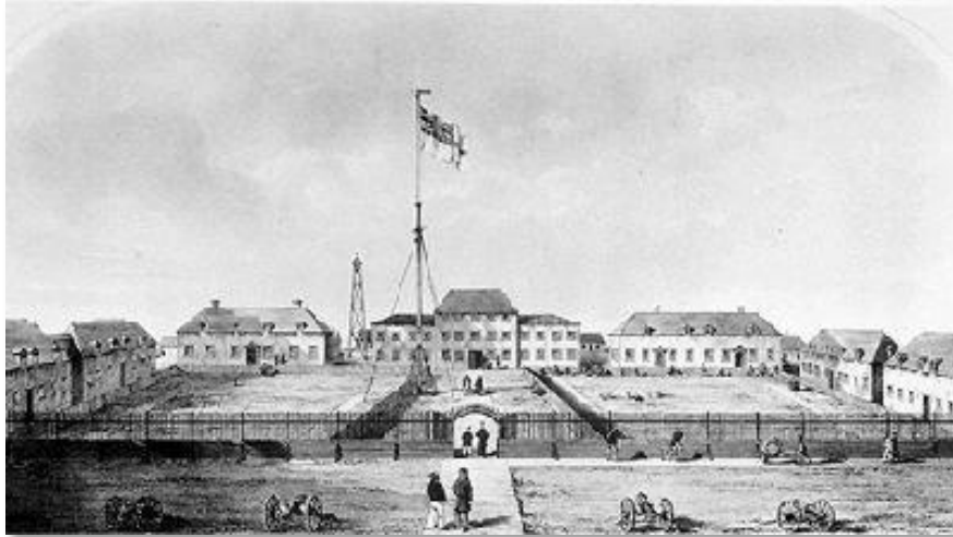
York Factory at Third Location
